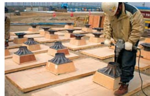
Fixing of casting at recess former
