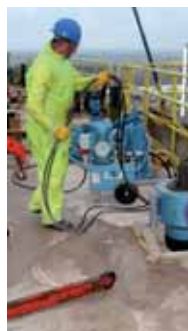
Stressing at the buttresses Vertical stressing
