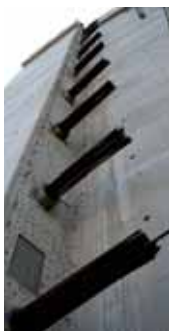
Stressing at the buttresses Vertical stressing
