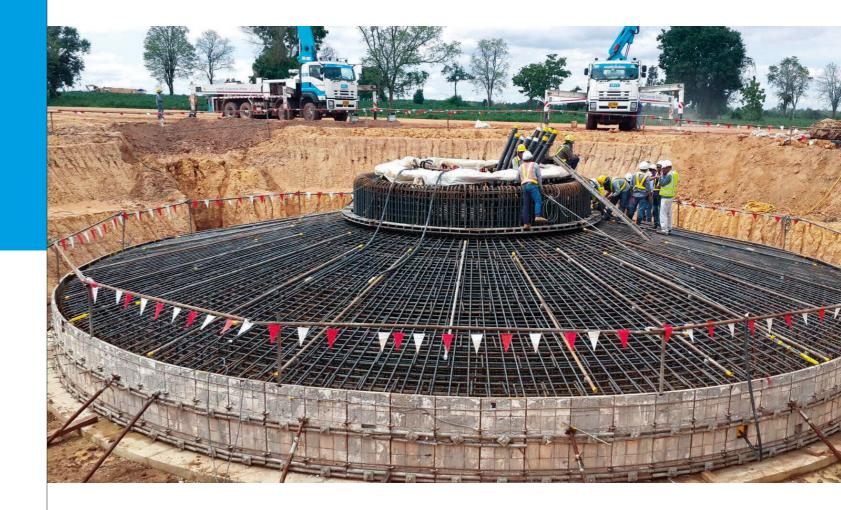
Construction of the foundations for 30 wind turbine generators as part of the Watabak Wind Farm, Thailand (2016).
