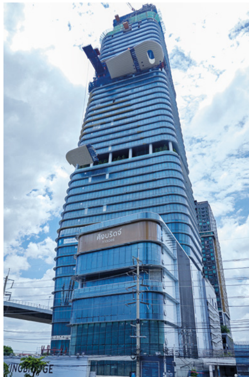
Precise coordination was required to slide the lifting frame and suspended floor truss 21m parallel to the building and 13m towards it.
