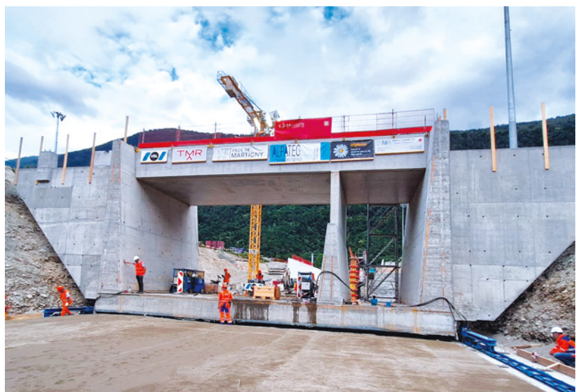
VSL performed the skidding of the box, which was built offline and had to be slid by 30 metres into its final position.
