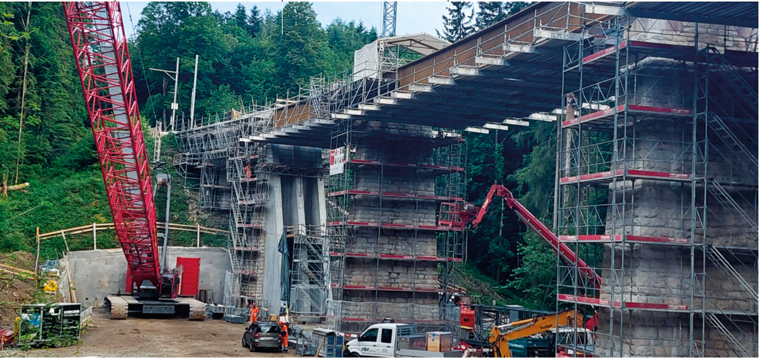
GEISSLOCH VIADUCT ON THE SOLOTHURN-MOUTIER RAILWAY LINE
