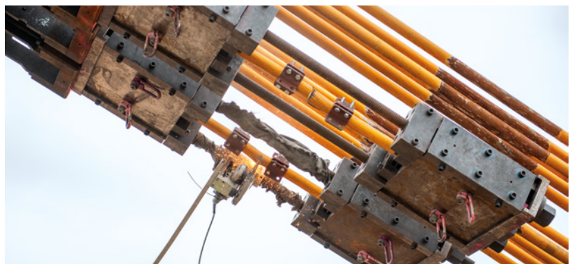
VSL replaced friction clamps with an innovative wedge clamp, forming a solid confining block within the de-tensioning assembly. This eliminates manual intervention, enhancing both safety and performance.
