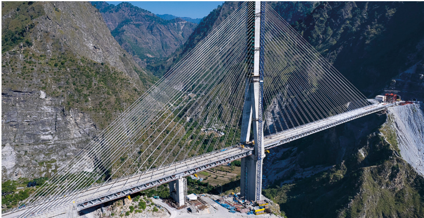
The new Anjikhad Railway Bridge carries the railway over a deep ravine between two tunnels. The main span is the longest cable-stayed span on Indian Railways.
