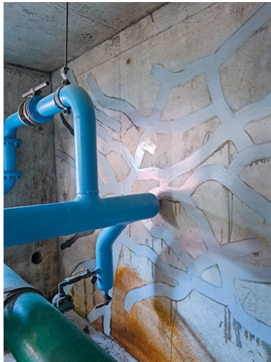
For the concrete repairs, VSL employed low-viscosity epoxy injections to address cracks and high-performance repair mortars for spalling areas.
