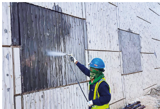
Micro-concrete allowed the damaged areas to be precisely targeted and repairs executed efficiently.
