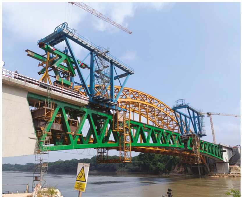
VSL's innovative solution involved the use of two SMU - 70 HL jacks to lift, launch, and lower the steel segments
