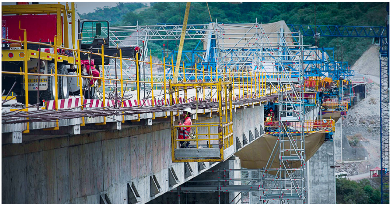
VSL Mexico oversaw the successful construction of the bridge deck, including reinforcement installation, concrete pouring and post-tensioning execution.
