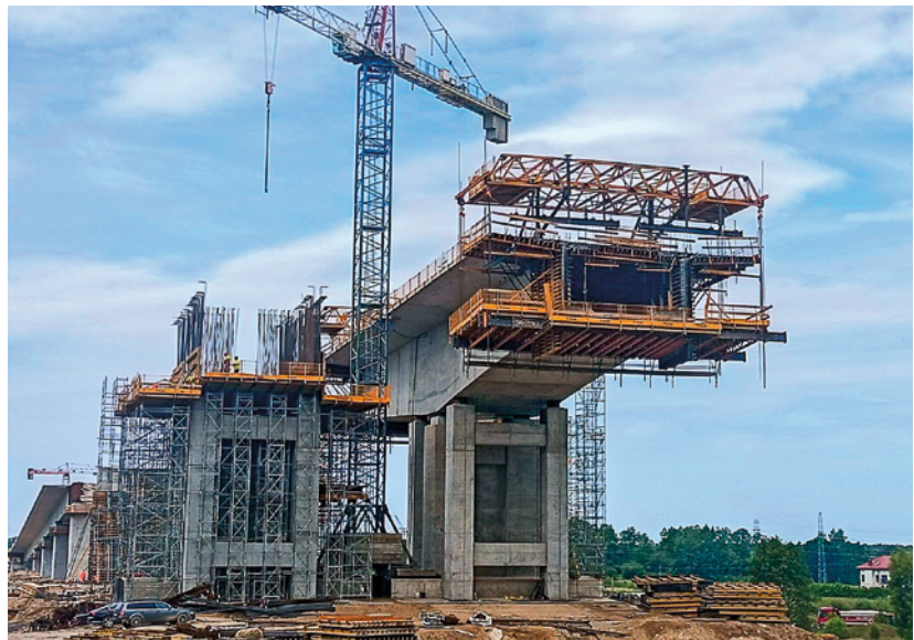
The balanced cantilever method was used to build a 390-metre-long section of each bridge, including a maximum span of 130 metres across a railway line.
