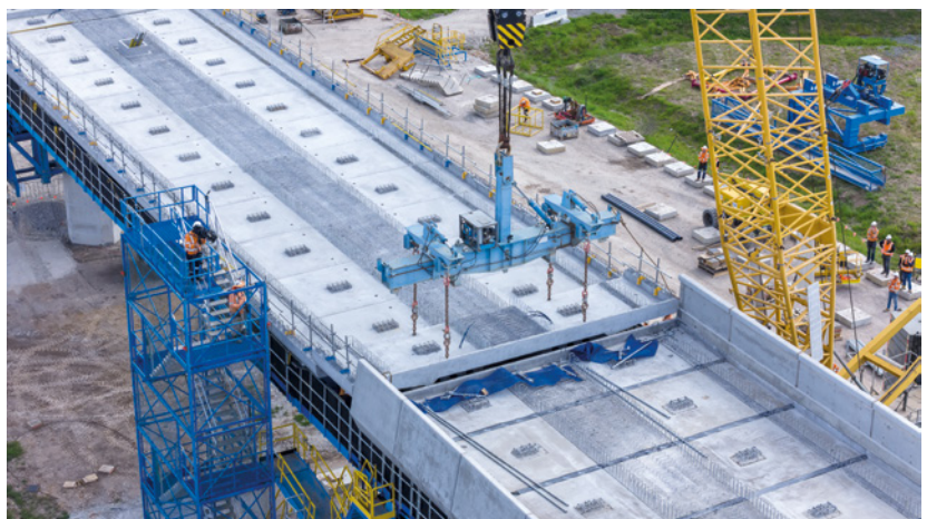
The team developed a C-hook to lift standard viaduct segments, preventing segment movement and eliminating the need for riggers to work at height or handle heavy rigging equipment manually.
