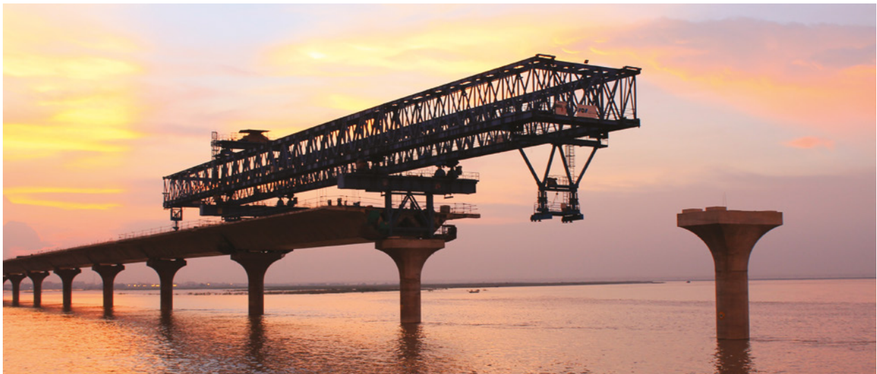
VSL's innovation in designing and supplying segment pre-casting cells, coupled with the implementation of the GEOCON geometry control software for the short line method, revolutionised the project.
