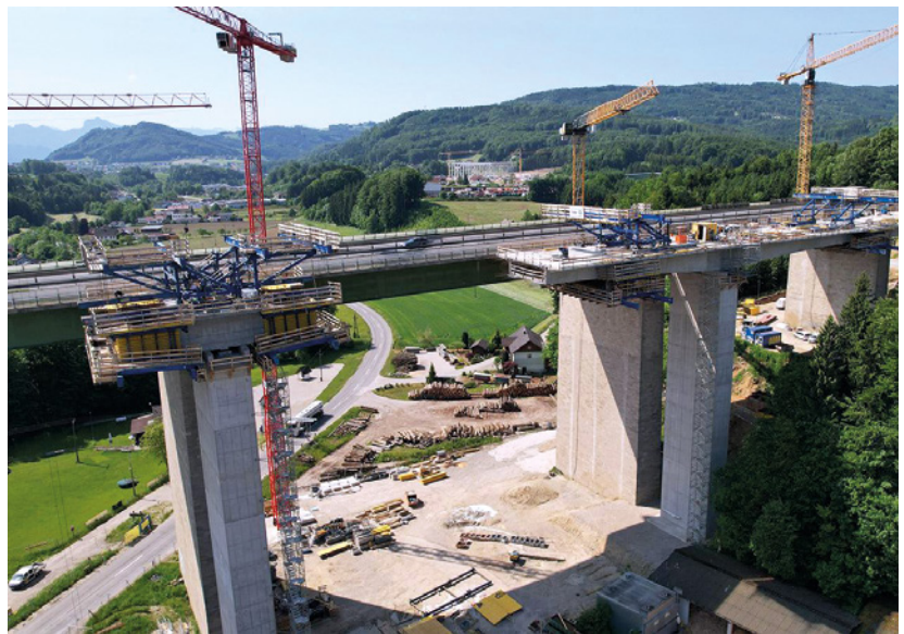
VSL Switzerland supplied and installed the post-tensioning system for the bridges.
