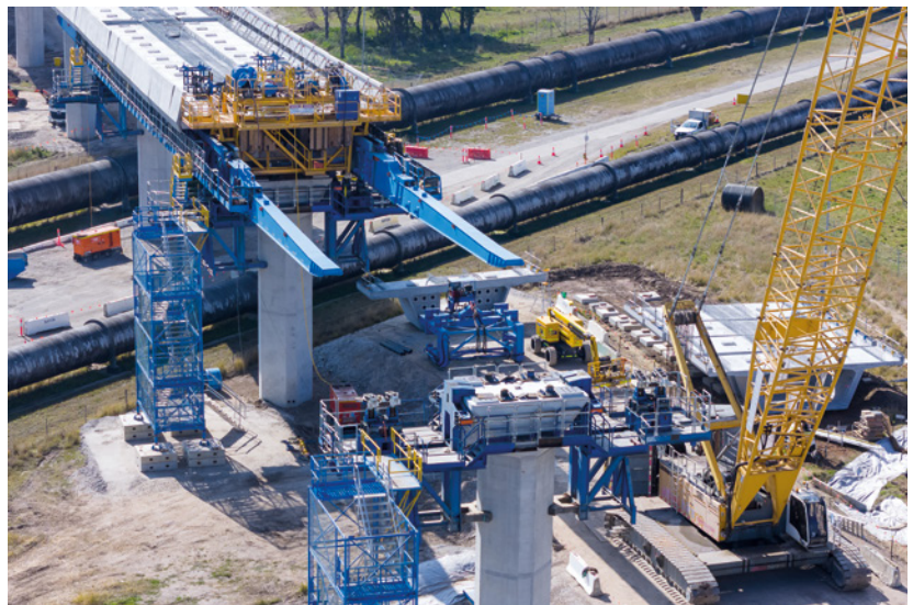
To address construction needs efficiently and minimise impact at ground level, VSL employed a combination of falsework and an underslung temporary beam (UTB). The UTB was the primary method of erection, offering a faster cycle time and reducing ground impact.
