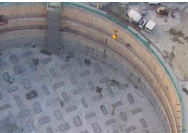
Top | Asia World Expo - Hong Kong Bottom left | Friction barrettes and diaphragm wall at ICC Tower - Hong Kong Bottom right | Underground car park
