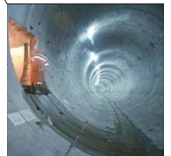
Ground improvement by grouting or soil freezing techniques for the construction of cross passages and tunnel adits.
